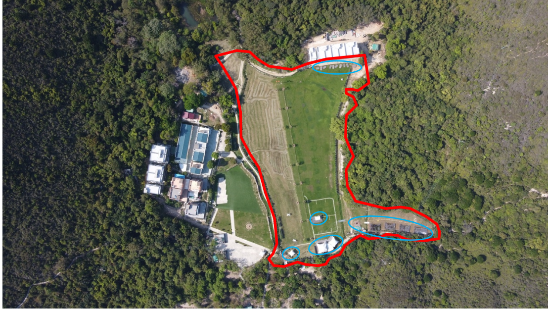
Figure 1 According to our recent site observation in April, some structures and construction materials (circled in blue) still scattered at northern and southern periphery of the application site (marked in red)
